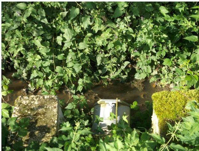
**PHOTOGRAPHIE 16 : CLAPET SUR TROP PLEIN DU POSTE DE RELEVAGE**
