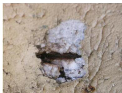
**PHOTOGRAPHIE 11 : FISSURE AVEC ACIER APPARENT CORRODE SUR LE GENIE CIVIL DU LIT BACTERIEN**
