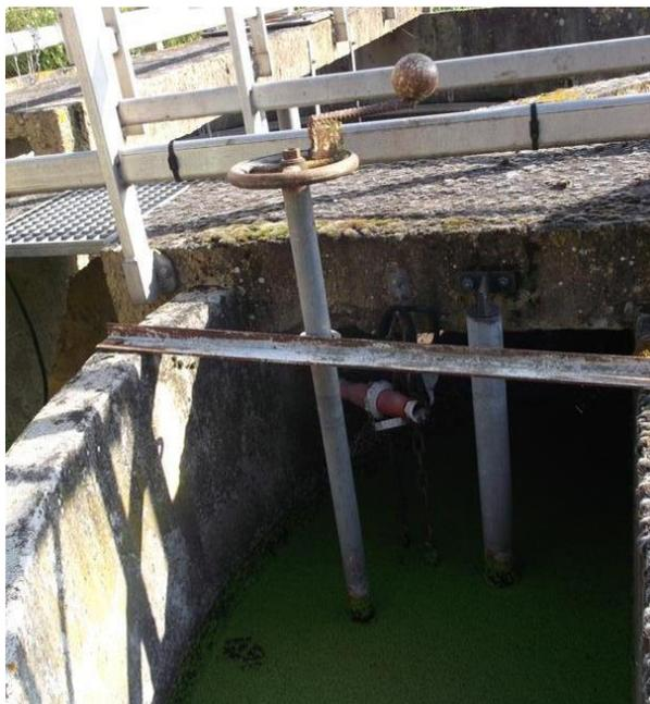
**PHOTOGRAPHIE 13 : VANNE D'ISOLATION DU PUIS A BOUES + POMPE DE RECIRCULATION DES BOUES**
